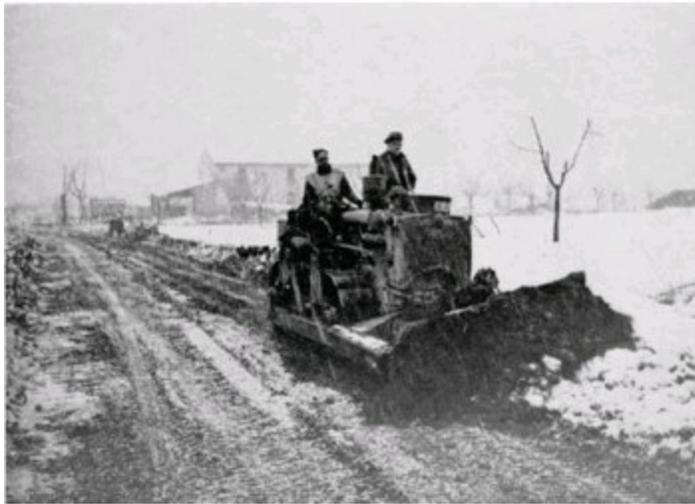
**A 27 Mechanical Equipment Company angledozer clears a highway in the [Faenza](#) sector**
