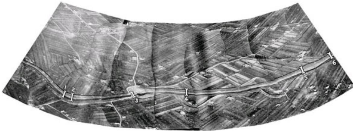
Approximate positions of bridges built by New Zealand engineers over the Senio River, 9-10 April 1945. The bridges are: 1. Raglan low-level; 2. Raglan high-level; 3. Scissors bridge; 4. Seymour low-level; 5. Woodville low-level; 6. Woodville high-level
